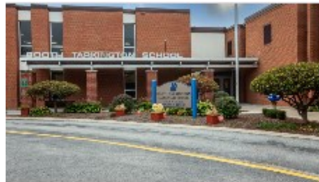
Tarkington Elementary School
